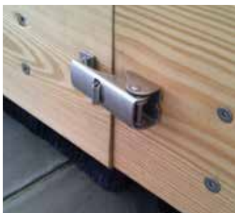
Simple and secure - quick release fastening
