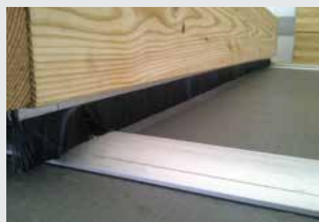
Brushes to perimeter to reduce debris entry
